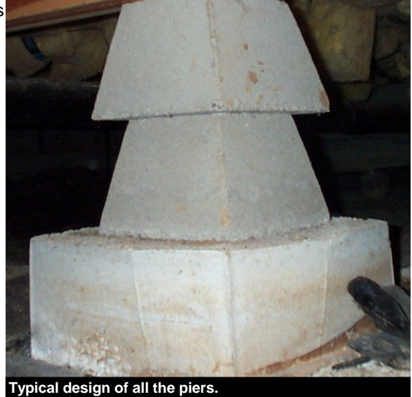
Typical design of all the piers.
